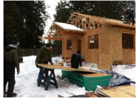
January 8: Progress on House 33
